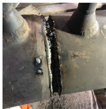
Fig. 4. Arc gouging results for defective weld. Source: Images made by the authors
